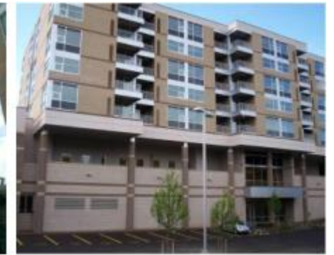
(b) five-storey CFS residential units built on an existing two-storey retail building
